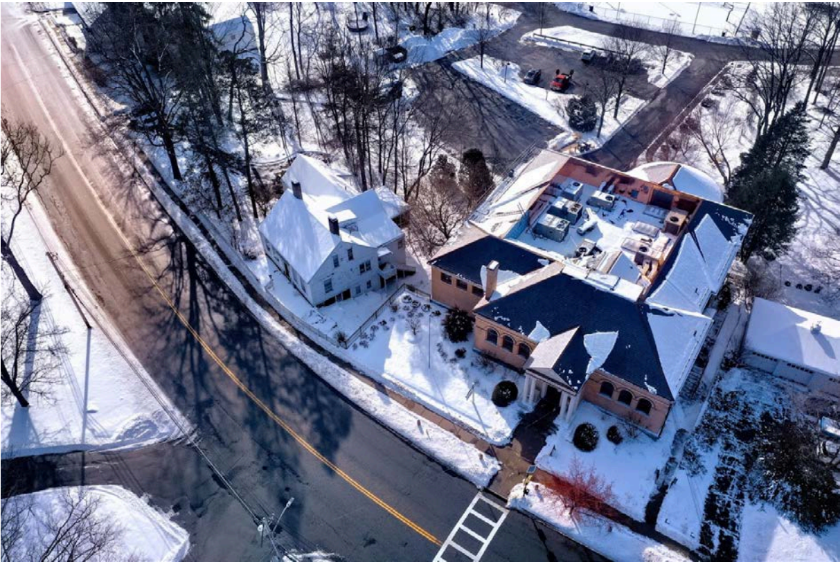
Photo: John Ellenberger, library roof nearly complete, Jan. 19, 2020
