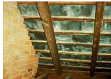
View of these slates laid on open sheathing shows that delamination and flaking are just as bad or worse on the underside of slates as on the exposed surface. This is why most slates cannot be flipped over for reuse.
